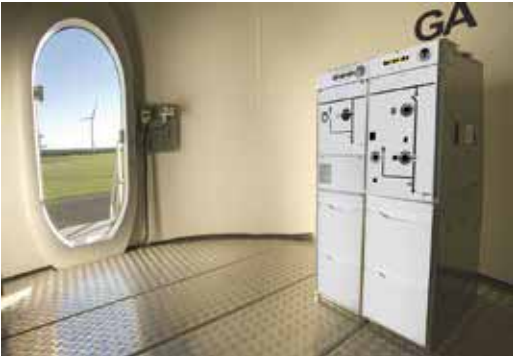
FBX-E in the mast of a wind tower, can be installed through a narrow door thanks to its compact size
