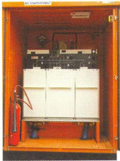
MV Compartment with Ring Master Type RMU
