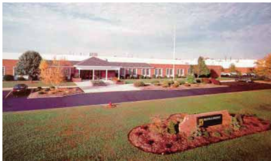
Square D facility in Oxford, Ohio U.S.A. is an ISO 9001 and ISO 14001 registered busbar trunking manufacturing facility.
